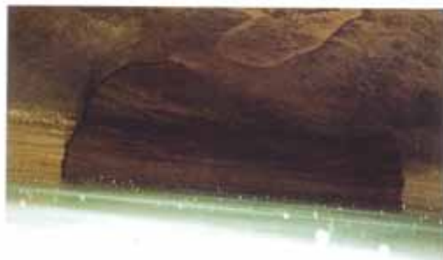
> The inner sections of the siphon (Photo Antoine Comaty)
