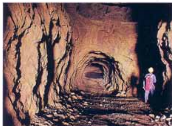
Photo 2 > One of the galleries in Marjaba mine (Photo Isam Bou Jawdah)
